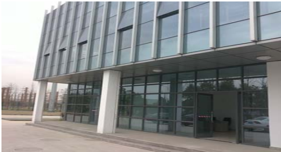
WuJiang MightYtek Plant
