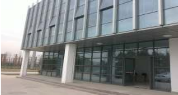
WuJiang MightYtek Plant
